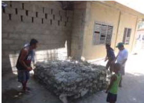
During the construction of ferrocement tank in Sagasa Island, Bien Unido, Bohol.
