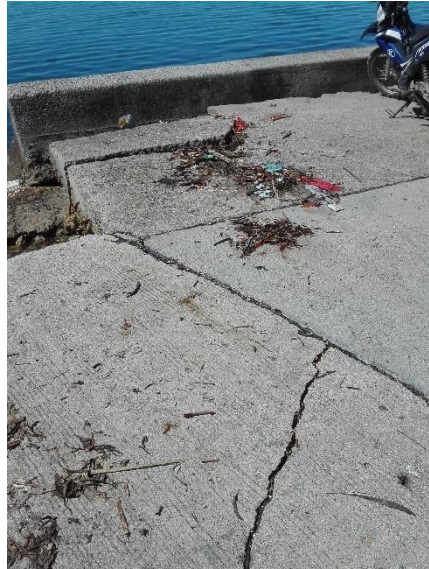
Figure 14. Cracks within the boardwalk created by the Earthquake.
