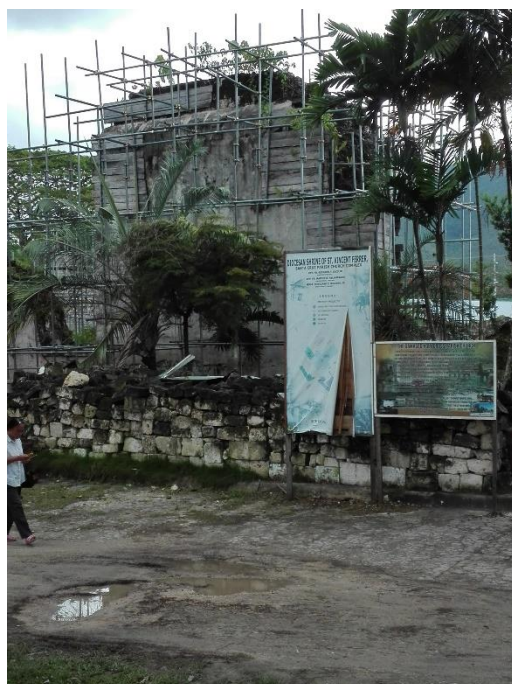
Picture 3. The remaining walls of the church. The construction withstands the walls of breaking down even more.
